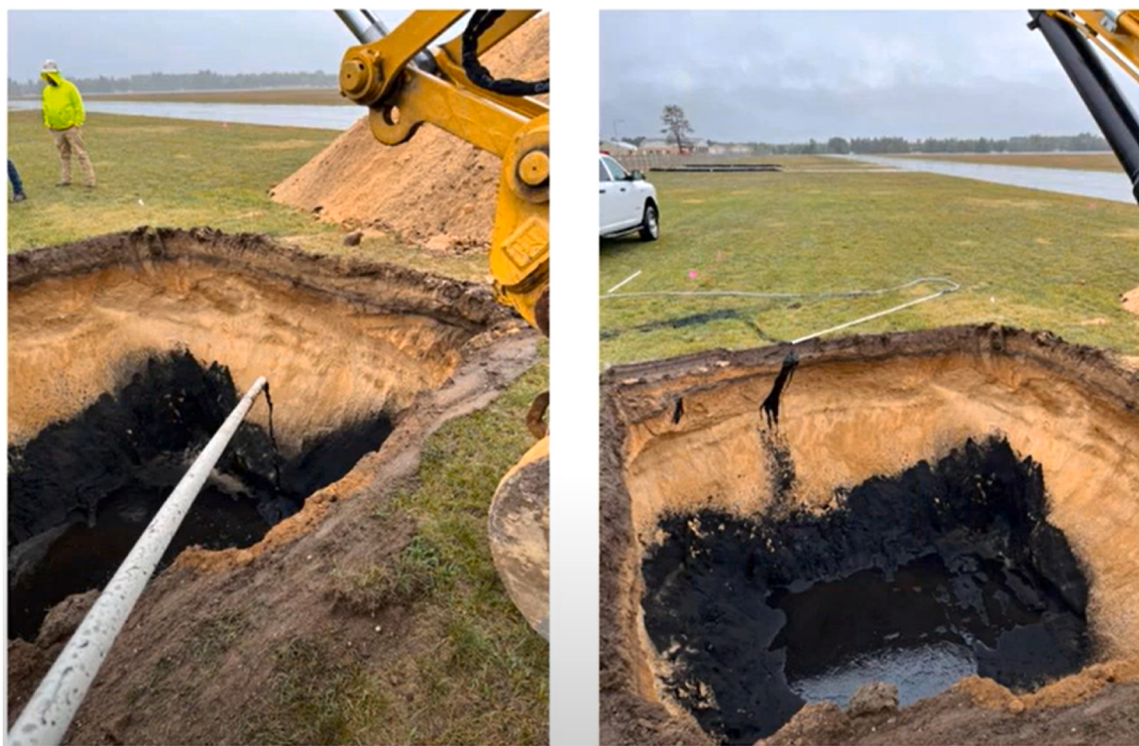
Fig. 6. CAC-enabled in situ remediation of PFAS-impacted vadose zone soil. Source: REGENESIS.
